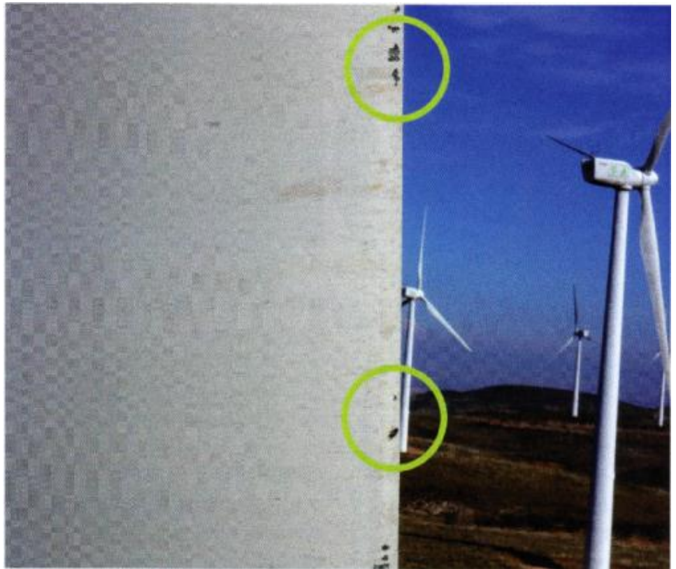
Leading edge damage, in detail, photographed by the EOL6.
